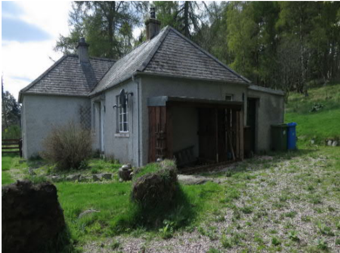
Existing bungalow to be demolished
